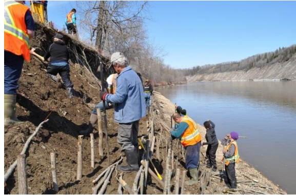
Soil bioengineering along the river
